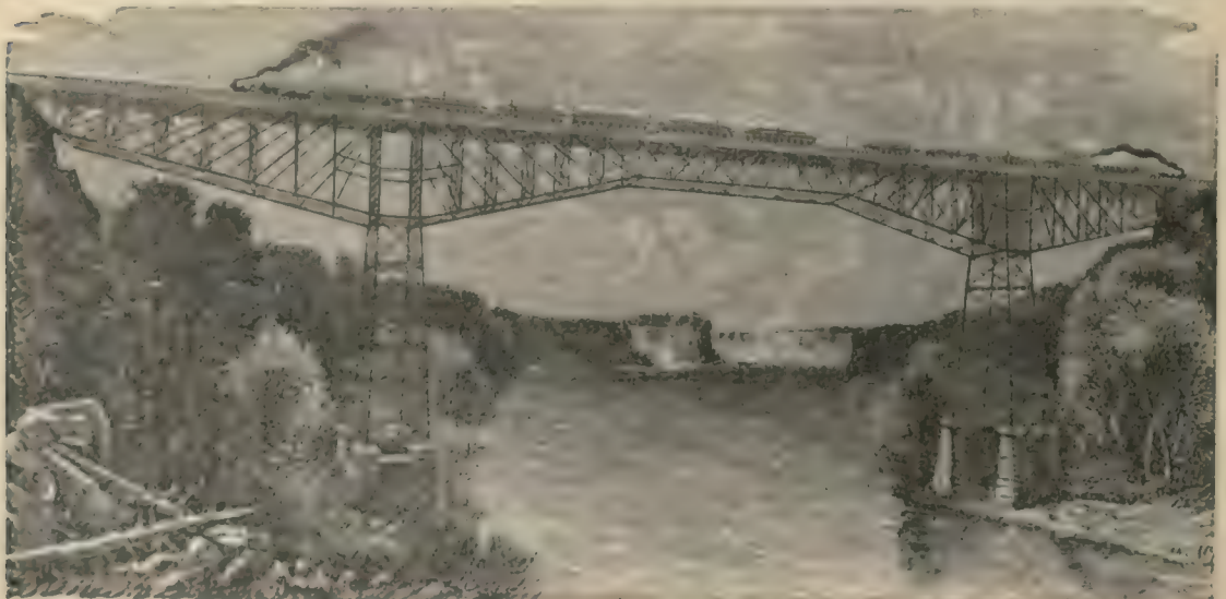
Cantilever Bridge over the Gorge at Niagara Falls.
